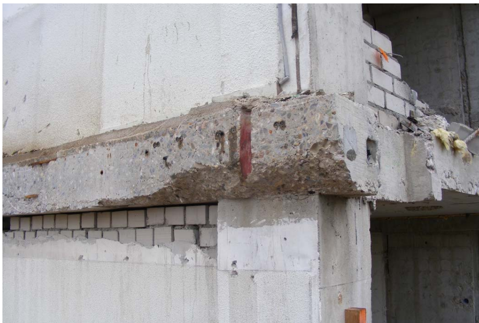
Foto 12: 2 e verdieping, randstrook op as e.
