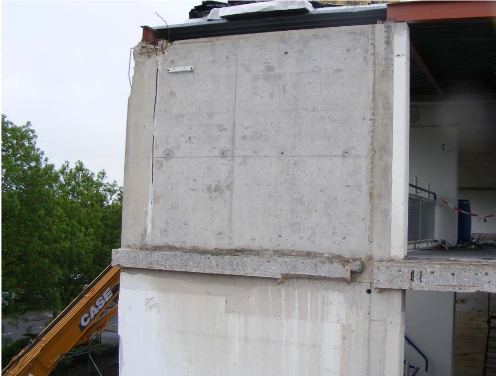
Foto 20: 3 e verdieping, tussen as a en c.
