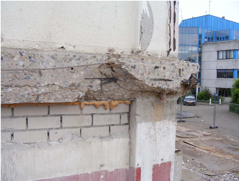
Foto 9: 1 e verdieping, randstrook op as e.
