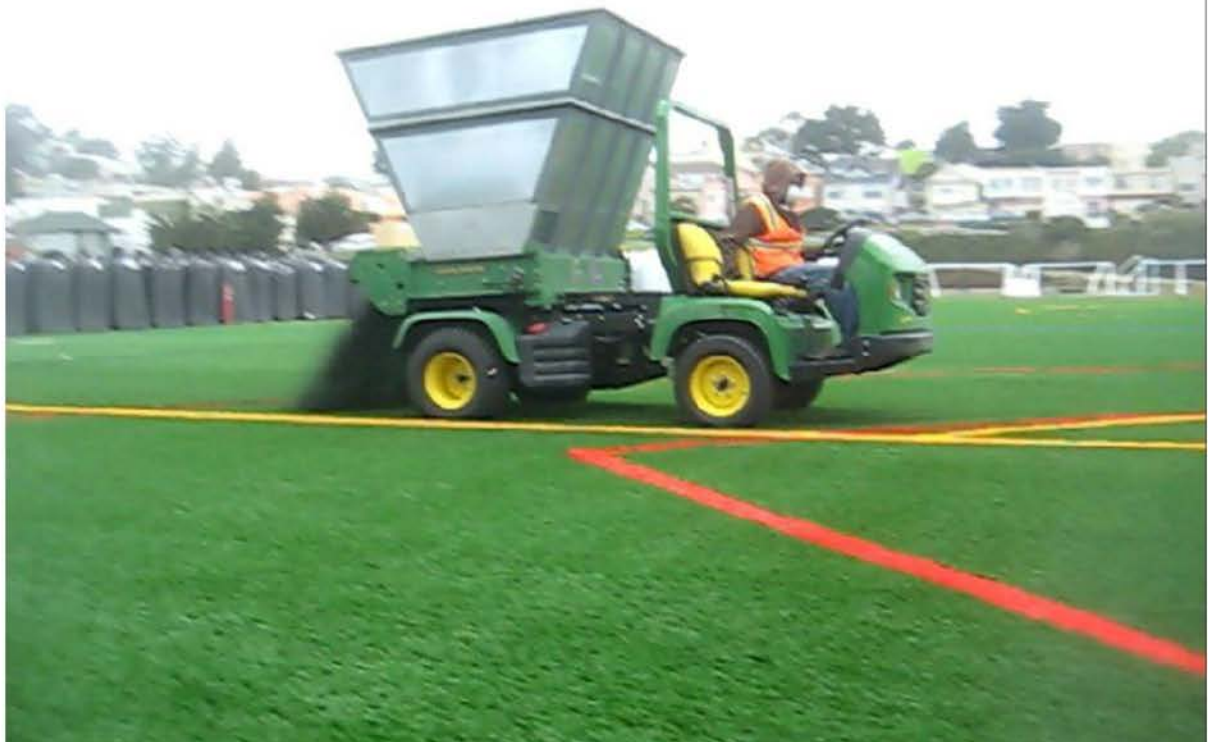
Figure 3.2 Semi-mechanised application of infill
