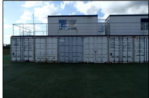
Bebouwing in plangebied.
